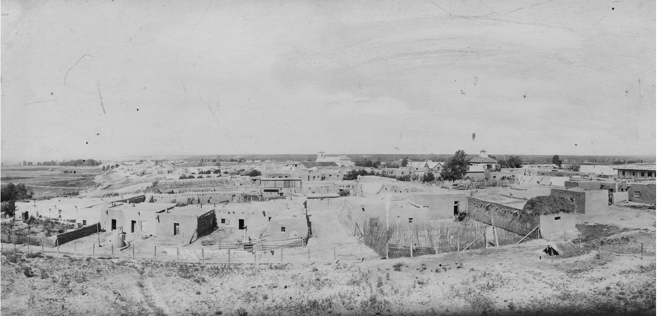
Figure B-4. Early photograph of Taos looking east, c. 1900. The Guadalupe Church, center background, is the tallest building, the Plaza is the treed space in front. (Town of Taos)
