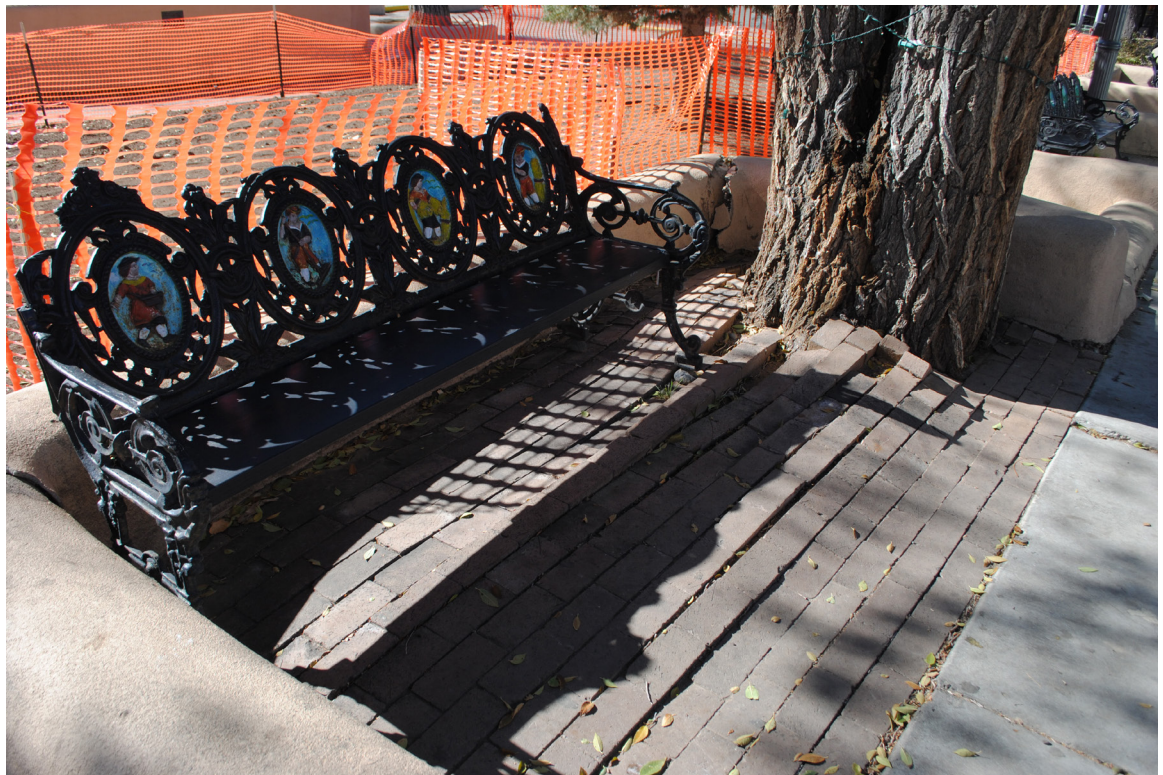
Figure 3-21. Several styles of benches exist in the Plaza, and paving is in poor condition throughout. (Mundus Bishop 2015)
